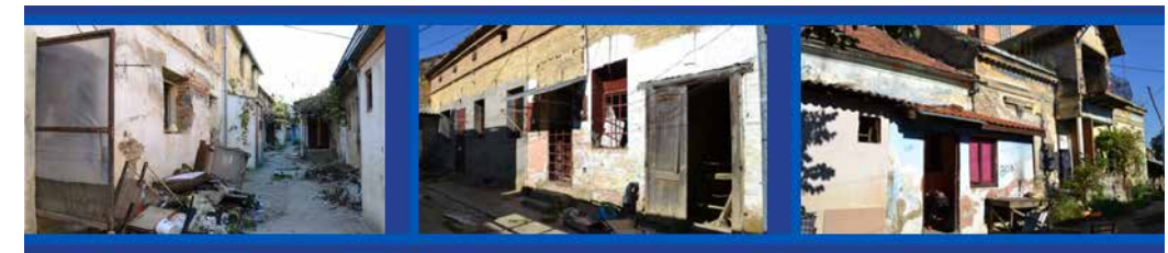
Picture 2. Examples of Roma families living in buildings not constructed for housing: 18 families living in abandoned warehouse (left), 12 families also living in abandoned warehouse (middle) and 14 families living in former City House (right), all in Obrenovac municipality, Serbia. Source: OSCE (2014).
